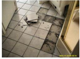
thus causing not only floor cracking but also joint adhesive failures in the roof and sidewalls. When the body flexes, the floor has a degree of twist, which in turn can cause the grout between the tiles to crack. After a period of time the grout can disintegrate leaving a wider crack and that is when everyone starts pointing fingers.
